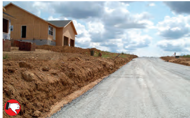
This residential management site shows poor management of bare soil areas. No erosion and sediment controls are present, and the grade on the existing slope is inadequate. Temporary or permanent seed, sod or mulch must be applied as soon as final grade is achieved. No slopes steeper than 3:1 are recommended.
