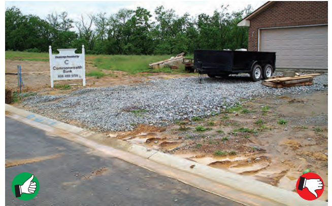
Rock sizing and placement look OK for a residential site, and very little mud appears on the pavement. The pad is a little thin, however, and it looks like some drivers are not using it—note track marks near curb. Adjacent soil areas need seed and mulch.
