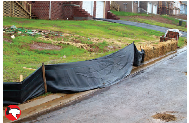
Poor installation of silt fencing, fair to good seeding. Silt fence must be trenched in along bottom and include wire backing. Straw bales are not approved as sediment barriers.
