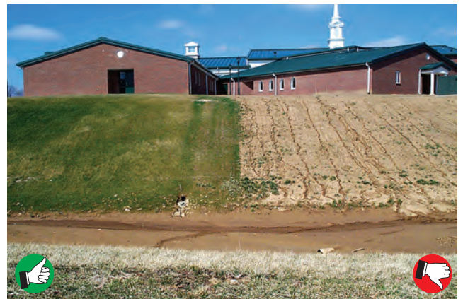
Erosion and sediment loss is virtually eliminated on seeded areas (left side). Rills and small gullies form quickly on unseeded slopes (right side).
