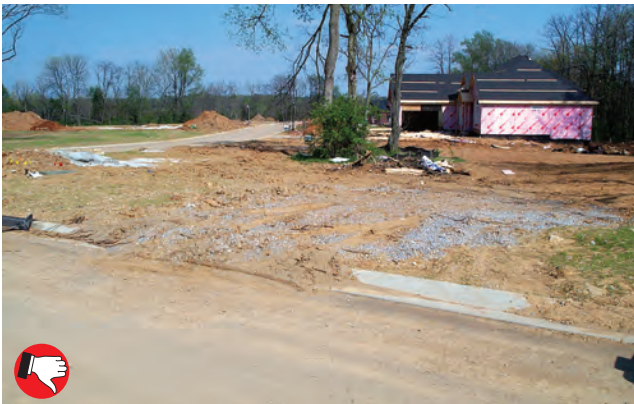
Poor construction entrance. Rock pad is poorly constructed; rock is too small. Use filter fabric under rock and larger sized rock, such as 3-5 inches. No mud should be tracked onto paved roads open for traffic.
